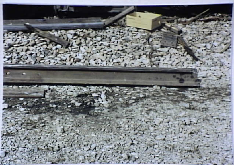
Photo 7. View of the West end segment of the 14 foot 11 1/2 inches "plug" rail
